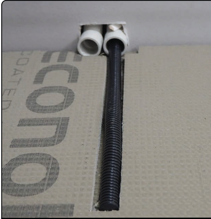
Push the supplied flexible conduit out into the channel in the floor. Ensure that the black cap is firmly in the conduit.
