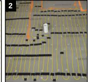
Plan out the installation Determine the location of the cable thermostat and floor sensor. calculate the available floor space (excluding floor mounted fixtures) and calculate the required cable spacing. Check you have all the required components.
